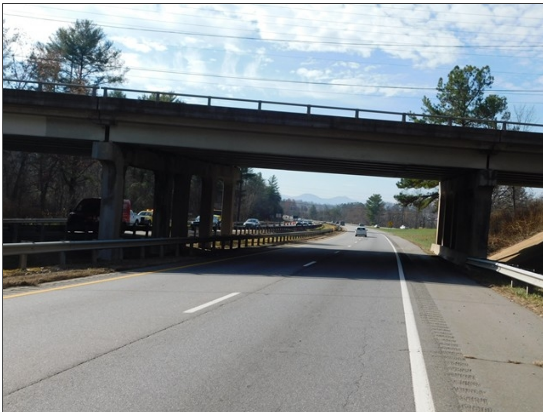
SPAN 3 OVER I-26 EASTBOUND
