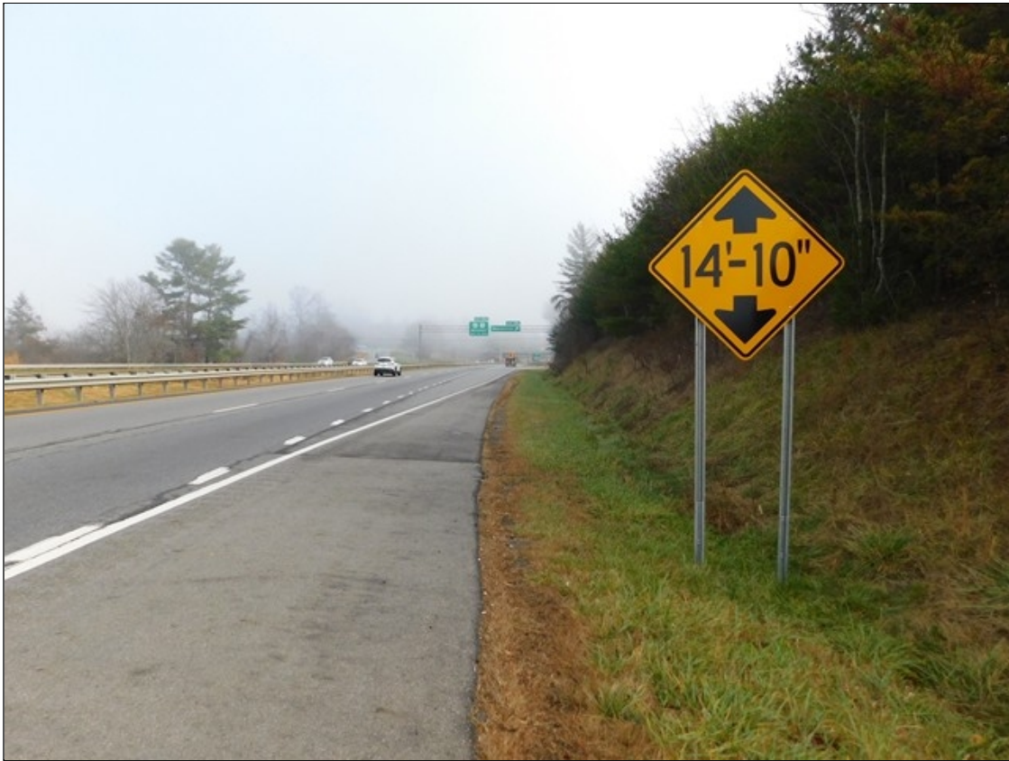
EAST APPROACH LOW CLEARANCE SIGN AT 600 FEET FROM THE STRUCTURE
