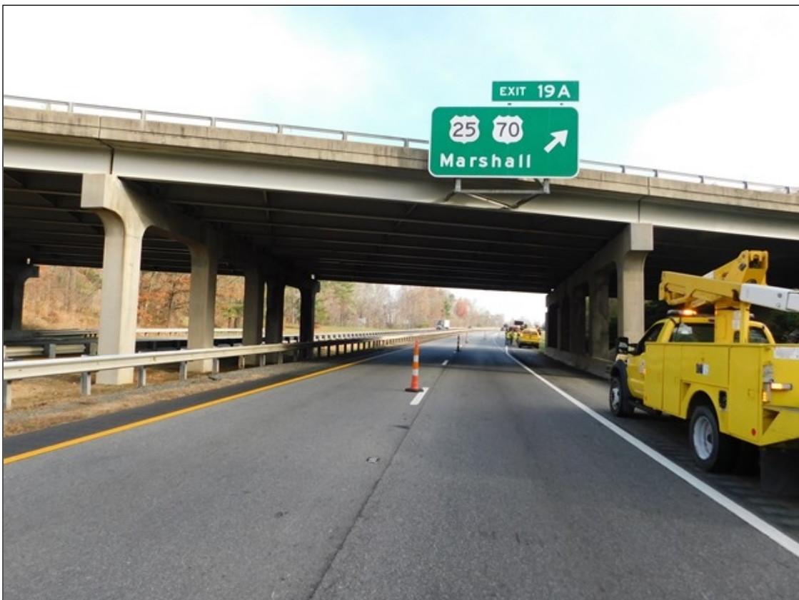
SPAN 2 OVER I-26 WESTBOUND
