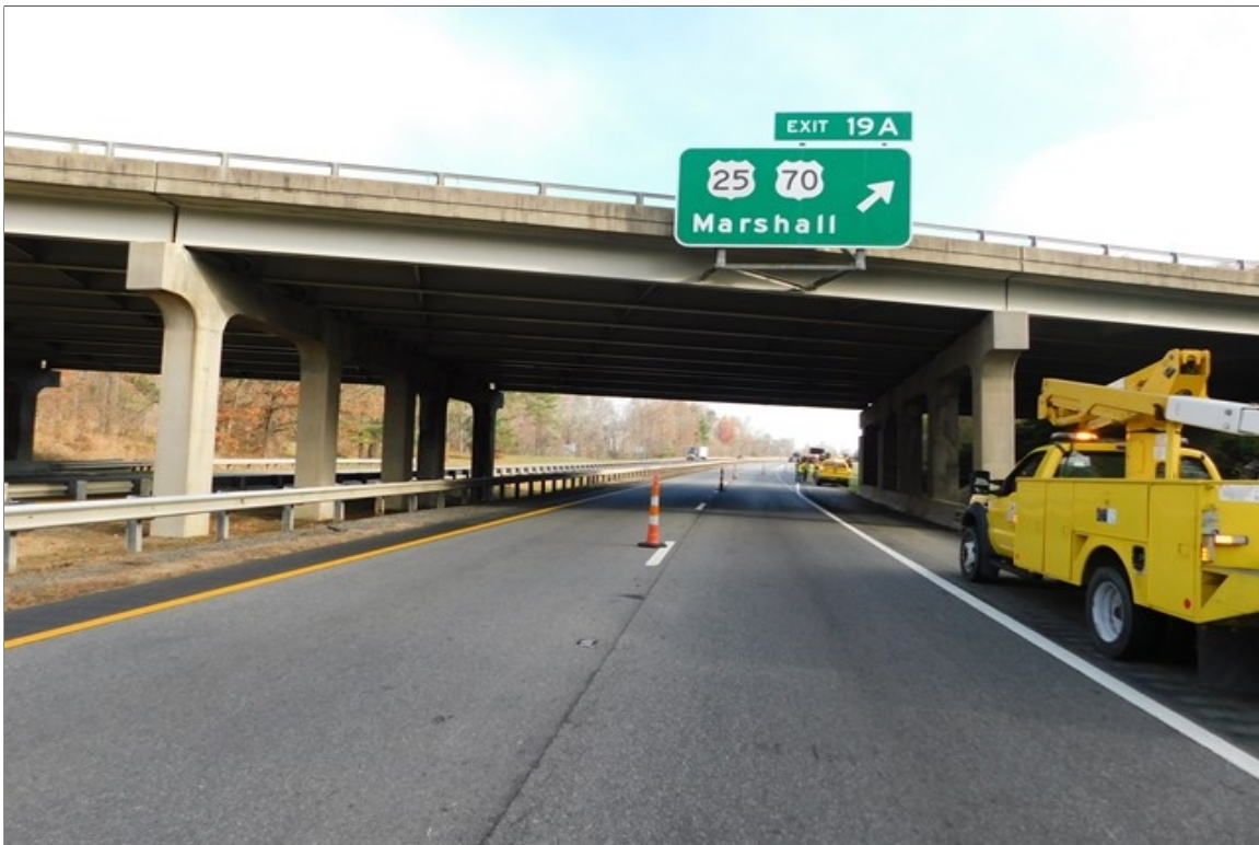
SPAN 2 OVER I-26 WESTBOUND
